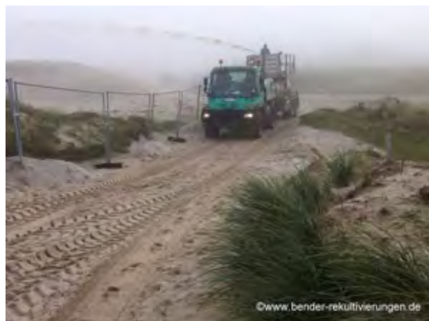
Surface stabilization for dust control at an industrial site using soil binding agents applied by a hydroseeder. Source: Bender GmbH & Co.KG.
