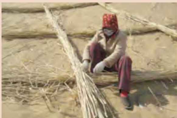
Initial stabilization of sand dunes using checkerboards
